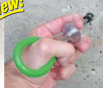
Insert into a properly-sized, cured concrete hole.
